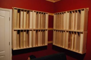
The installers field fabricated some Schroeder diffusers to help create a balanced and full sound in the small studio.
