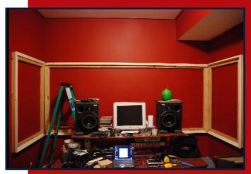
The picture above shows the Wallmate track installed on top of the 1" thick furring strips. This allowed the owner to use the 2" thick recycled cotton panels to achieve a desired result. The 2" thick panels have a better low-frequency response with regard to the 1" thick panels that are considered "standard".
