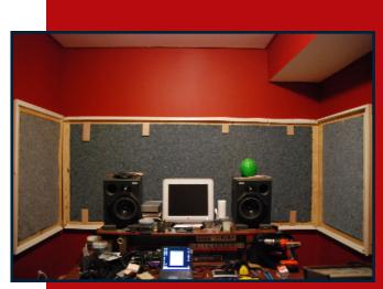
The Echo Eliminator was adhered to the wall with a construction adhesive. For this installation, the installers used some wood scraps to hold the panels in place – these were temporary to hold the panels until the adhesive dried.
