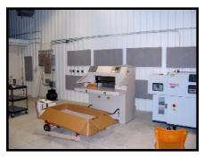
Based on the cubic volume of this room, fifty-six panels were installed. The panels were our 1" thick, #3 lb. density Light Gray Echo Eliminator™ which are made from recycled cotton fiber. They were installed onto the walls with construction adhesive. The customer had no problem installing themselves and decided to install the panels in a pattern which balanced the quantity through out the space.
