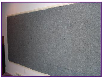
These pictures show the Wallmate™ track as well as the Echo Eliminator® acoustical cotton core as they are being installed. The tension of the fabric is pulled in all directions and stands slightly off the cotton to hide any seams between the acoustical panels. Ideally, we try to supply the cotton core as close to the color of fabric as possible.
