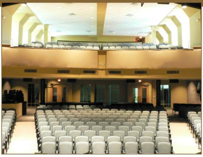
The choir and director at the new life church were getting a significant echo caused by the curved flat surface that made up the structure of the balcony. Because the building was brand new, they needed a decorative acoustical panel that would fit the curve of the large, flat reflective area.
