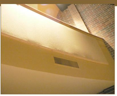
Because the building was so new, this customer did not want to adhere the cotton panels to the wall before they stretched the fabric - which is STRONGLY recommended. The concern was that they did not want to do anything that would have such a "permanent" affect on the room. After the fabric was stretched, it began to sag slightly, taking away the sharp borders of the track.
